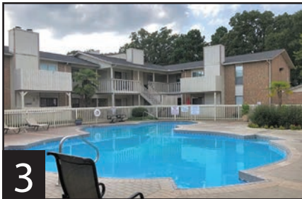
3 Richmond Oaks 2815 Richmond Road Texarkana, TX 75503
